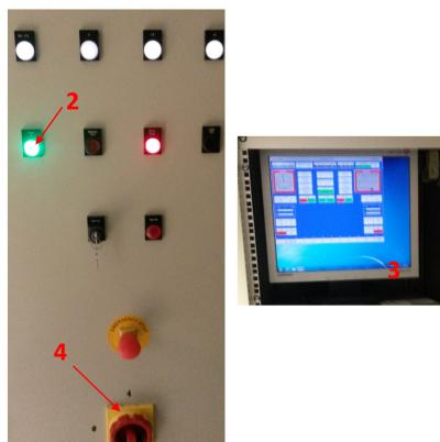
(Afterwards only UPS is still on and powers the communication lines (red LEDs, see picture below))
