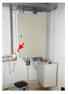
**3.** Keep the hand-control box switch on position II (where it should always be). It switches between control by handheld panel and a kind of raw mode (each motor can be controlled individually).
